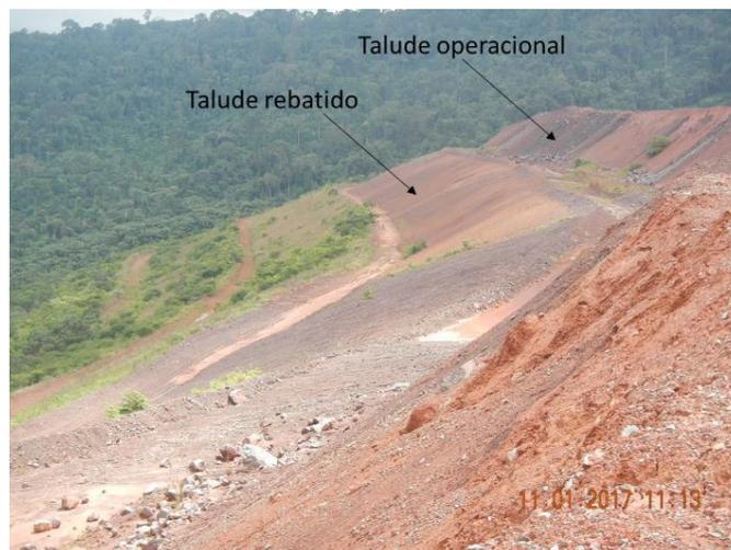
**Figura 8: Talude rebatido e talude operacional (Costa, 2018).**
