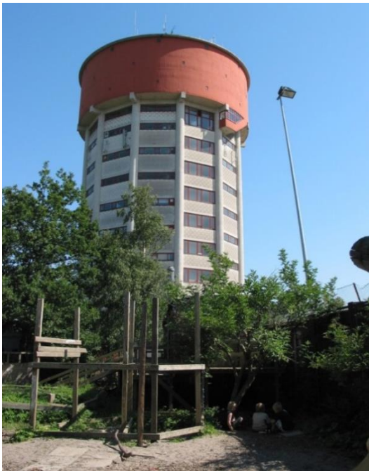
Figura 17 - Jægersborg Water Tower
